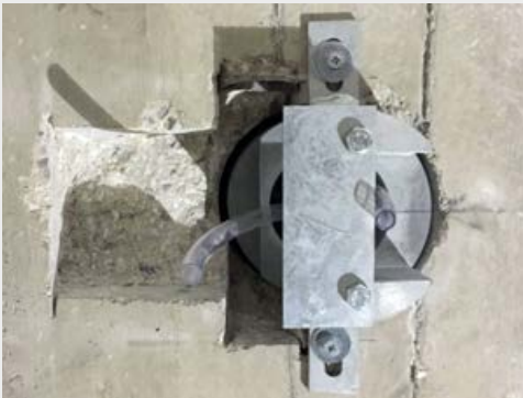
Step 2: Fitting the fixed and movable anchors
