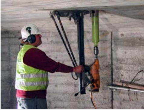
Step 1: Drilling for the anchors
