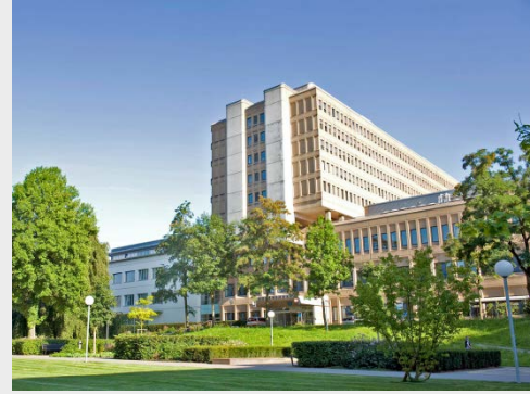
Earthquake strengthening Hospital Aarau, Switzerland
