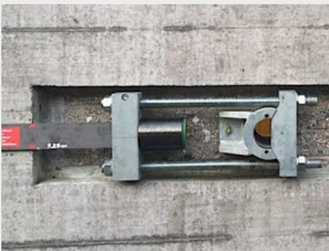
Step 3: Installing the CFRP plate at the anchors
