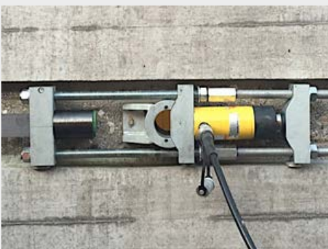
Step 4: Post-tensioning the CFRP plate
