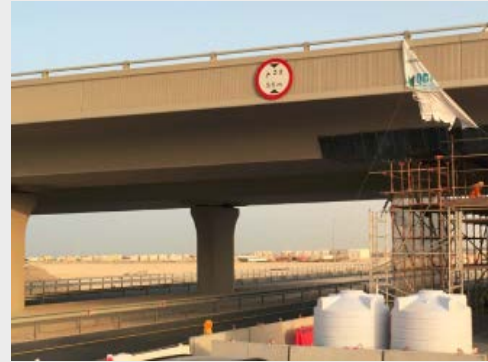
Bridge strengthening Bridge N29, Qatar
