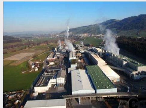
Beam strengthening Paper mill "Perlen", Switzerland
