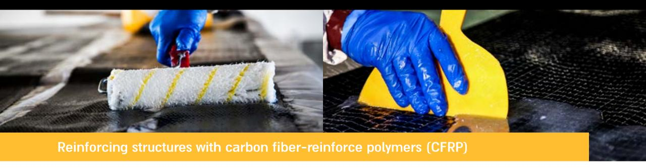
Carbon fibers belong to the family of composite materials. They are unique in combining exceptionally light weight with extreme tensile and structural strength.
